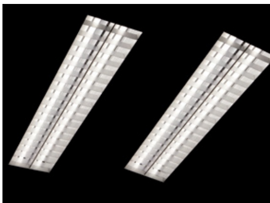
EUL in ceiling fixtures (1 on 1 replacement of fluorescent tubes)
